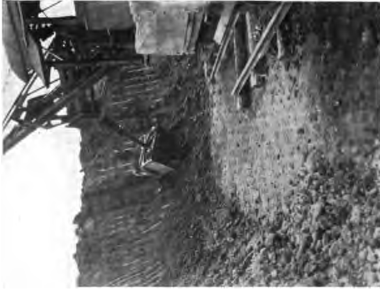
(A) Steamshovel excavating flood plain clay at Deacon, east of Lynchburg.
